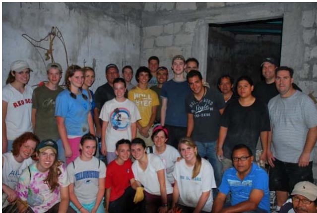
Service-learning is an important part of American Heritage School’s methodology. Recently, AHS students and parents helped to build homes in Veracruz, Mexico.
